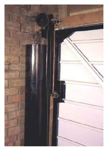
The counterweights were found on both sides of the door and made from pipe filled with steel washers, concrete, or stones. However, one-piece doors were hard to seal off from the outside elements which made them impractical in the colder climates of Canada. The poly-urethane insulated sectional door type quickly replaced one-piece doors in Canada and is now replacing one-piece doors everywhere in North America. Still, because of the simplicity in manufacturing a one-piece door, it
