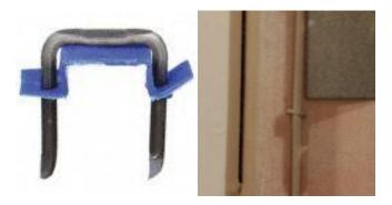
So, if you are stumped on what is causing Phantom operation/ you must check every staple used along the bell wire. A staple may be causing a short even if it looks fine. I would pull any staple that looks like it is pressing on the wire too hard.
