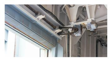
Of course, we must remember all garage doors have torsion type springs that are used as counterweights to help move a door up and down. Most people underestimate the power in the garage door springs and firmly believe the motor does all the work. I estimate the torsion springs are responsible for 75% of the heavy lifting. The operator is only a replacement for a person's arm and permits remote operation.
